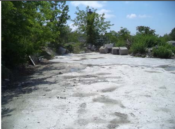
Photo 3: Southeast area of the platform. This area is mostly covered in concrete.
