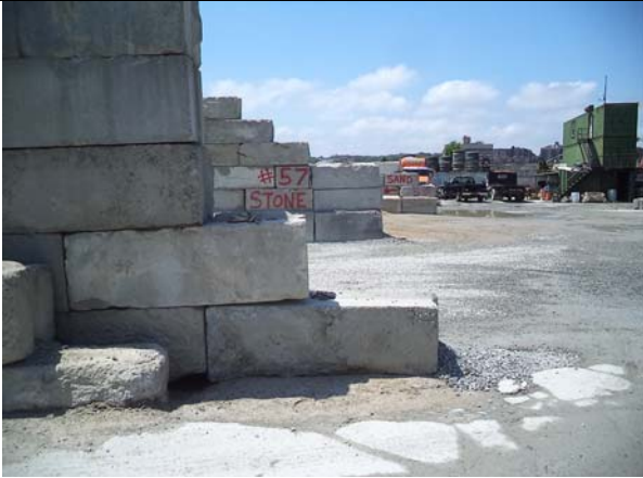
Photo 19: View of the southern portion of the Fordham Road Concrete.
