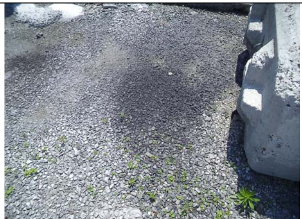
Photo 6: An area of discoloration at the southwest corner of the platform
