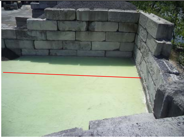
Photo 7: A shallow pool of unknown liquid (possibly concrete wash-out) at the southwest corner of the Site. The approximate Site boundary is shown as a red line.
