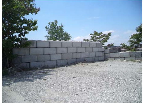
Photo 10: The northern wall of the platform.
