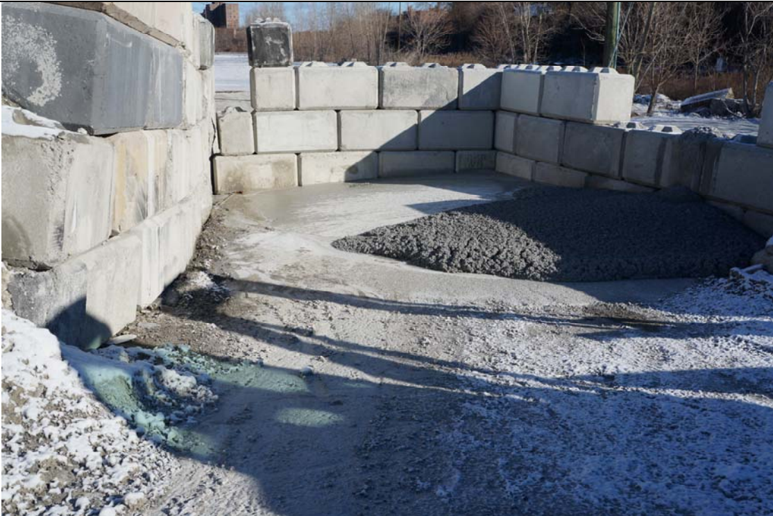
PHOTO 8: TRUCK WASHOUT AREA (TYP.)
