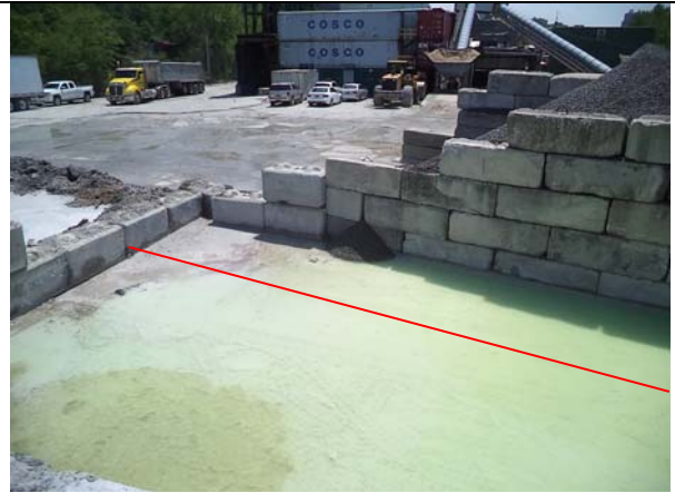
Photo 8: A shallow pool of unknown liquid (possibly concrete wash-out) at the southwest corner of the Site. The approximate Site boundary is shown as a red line. Fordham Road Concrete is beyond.
