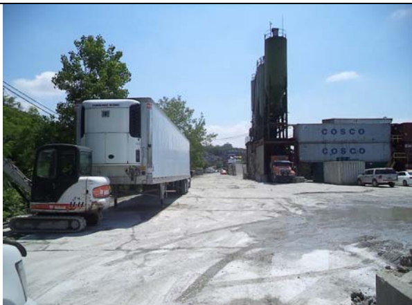
Photo 17: View of the southern part of the Site (Exterior Street) from the north.
