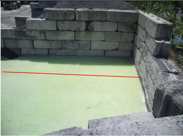
Photo 7: A shallow pool of unknown liquid (possibly concrete wash-out) at the southwest corner of the Site. The approximate Site boundary is shown as a red line.
