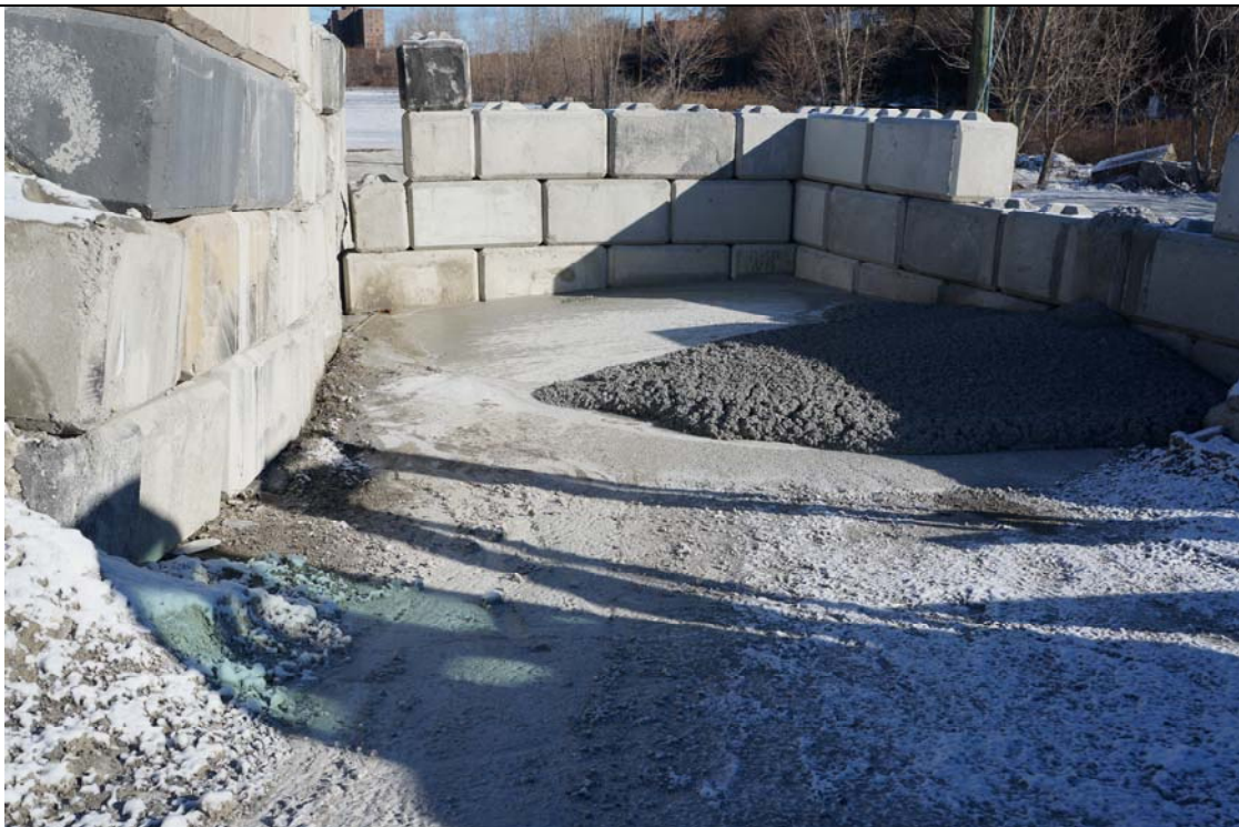
PHOTO 8: TRUCK WASHOUT AREA (TYP.)
