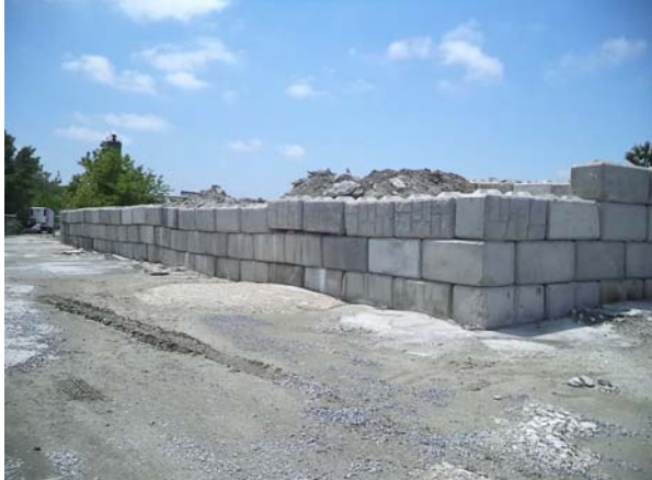
Photo 1: Eastern side of concrete block wall enclosing the platform at the southern end of the northern part of the Site. The entrance to the northern part of the Site is shown to the left of the wall.
